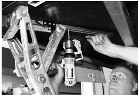
*Pilot-drilling for the last two fixing screws.*
